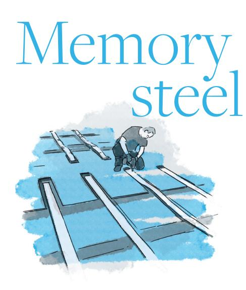
Memory steel, also known as shape memory alloy, is a unique material that can 'remember' its original shape and return to it when heated. This makes it more resistant to large amounts of strain, making it perfect for reinforcing structures.
